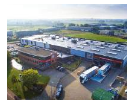
Raalte, The Netherlands
